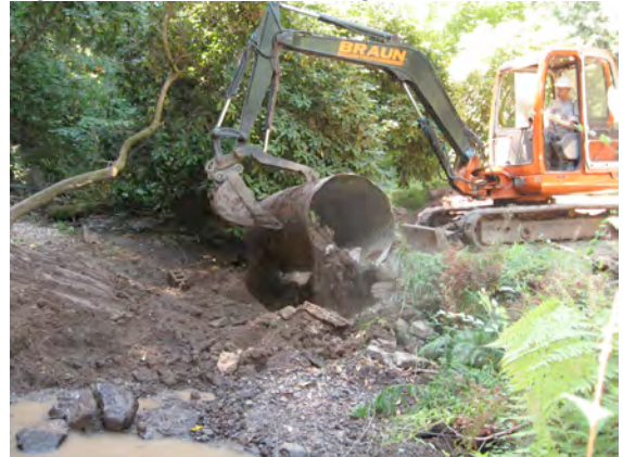
Figure 9: Construction to get rid of a culvert
