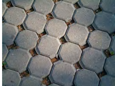
Figure 6: An Example of Porous Paving
