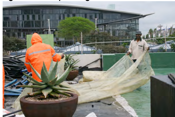
Figure 9: Waterproofing Roof Garden
