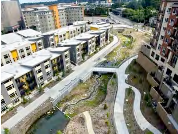
Figure 11: Finished stream daylighting project
