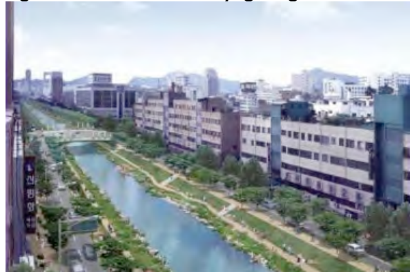
Figure 2: After stream Daylighting
