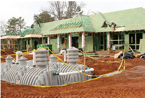
Figure 5: Cistern Installation
