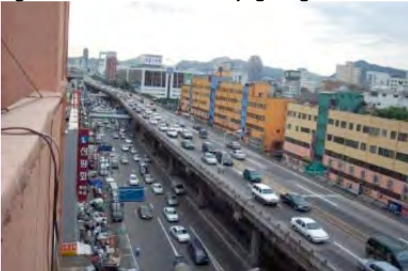
Figure 1: Before Stream Daylighting
