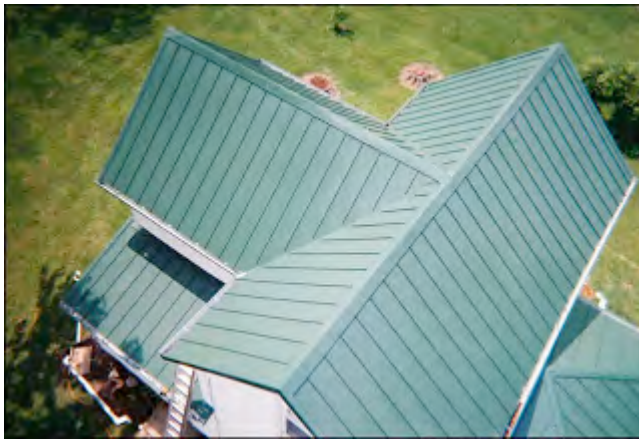
Figure 7: A Typical Residential Roof
