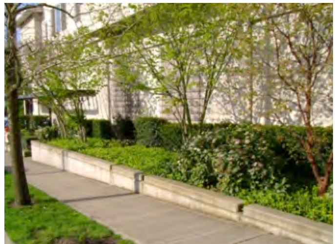
Figure 4: Example of Stormwater Planter
