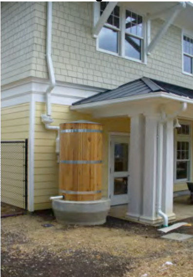
Figure 1: A Small Cistern for Residential Usage
